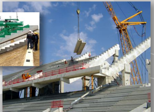
Handling precast elements
