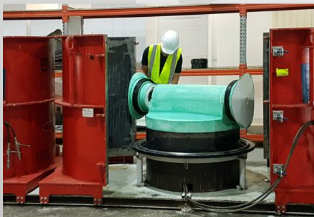
Coating / Connection of hole former
